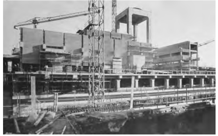
Fig. 154. Submarine Refit Complex, view from the west (January 1977). TNA, CM 20/64 (1976–77). PSA: Devonport: Works Projects. Photograph albums. Nuclear Submarine Refit Complex book no. 4. Reproduced with the permission of The National Archives.
