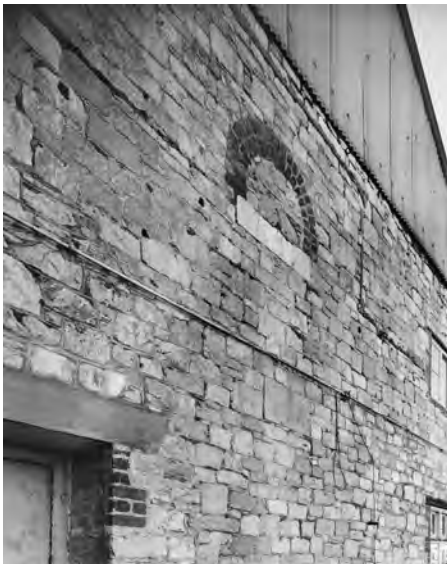
Left: Fig. 68. BB96/03859. Devonport South Yard South Smithery (S126) photograph detail of evidence of the line shaft on the north side of central building (29 Feb 1996). ©Crown copyright.HE.
