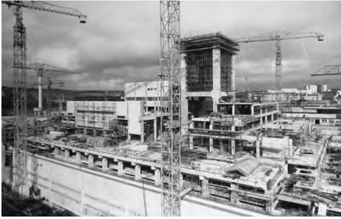
Fig. 153. Submarine Refit Complex (September 1976). TNA, CM 20/64 (1976–77). PSA: Devonport: Works Projects. Photograph albums. Nuclear Submarine Refit Complex book no. 4. Reproduced with the permission of The National Archives.
